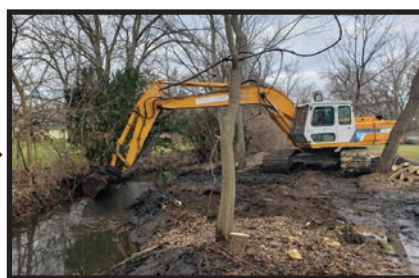
T ASD removes debris that was causing water to collect and breed mosquitoes.
