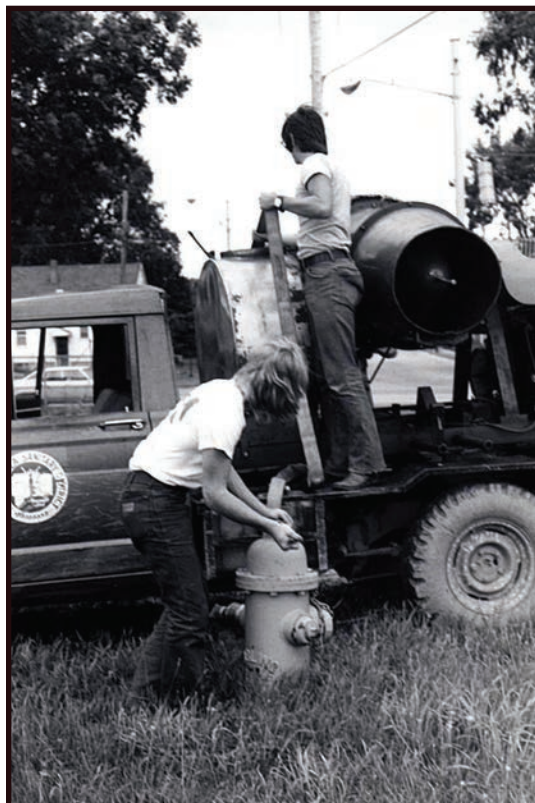
TASD employees add water from a hydrant to a mix for a product.
